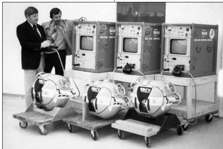
Drew Michel (with controller), of Taylor Diving, accepts three Hydro Products RCV 225 from Chuck Strickland. These were the first ROVs used in the Gulf of Mexico.
